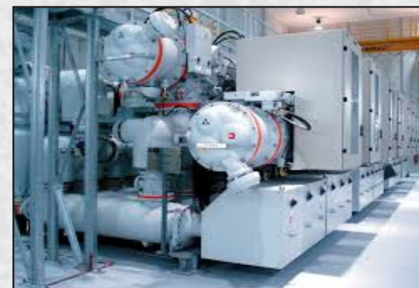
Gas Insulated Switchgear 132KV,220KV,400KV
